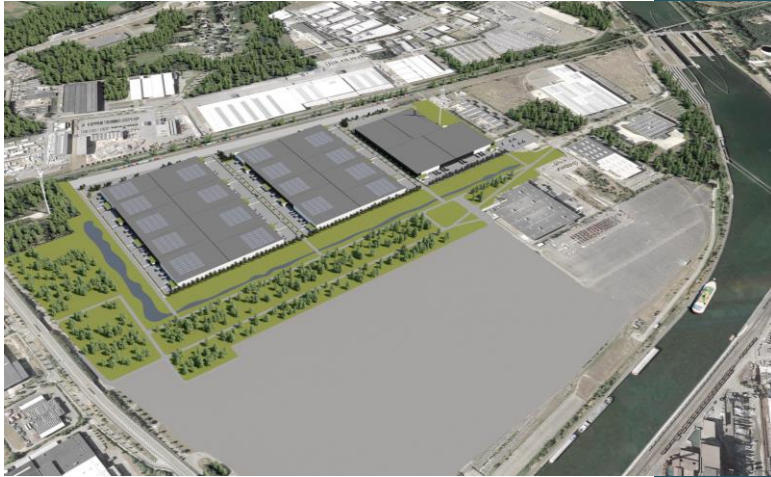
Genk Green Logistics Redevelopment zone B
